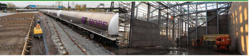
Six, 3,000 tonne storage cells were constructed using complex steel frames and raft slabs for the bulk store and a portal frame for the 2,950m² bagging warehouse, with 700 pre-cast concrete units being installed to form the cement store cells. Piling works took place with the installation of 1,500 fully reinforced pre-cast driven concrete piles, installed to depths of 9m using two hydraulic drop-hammer piling rigs.
